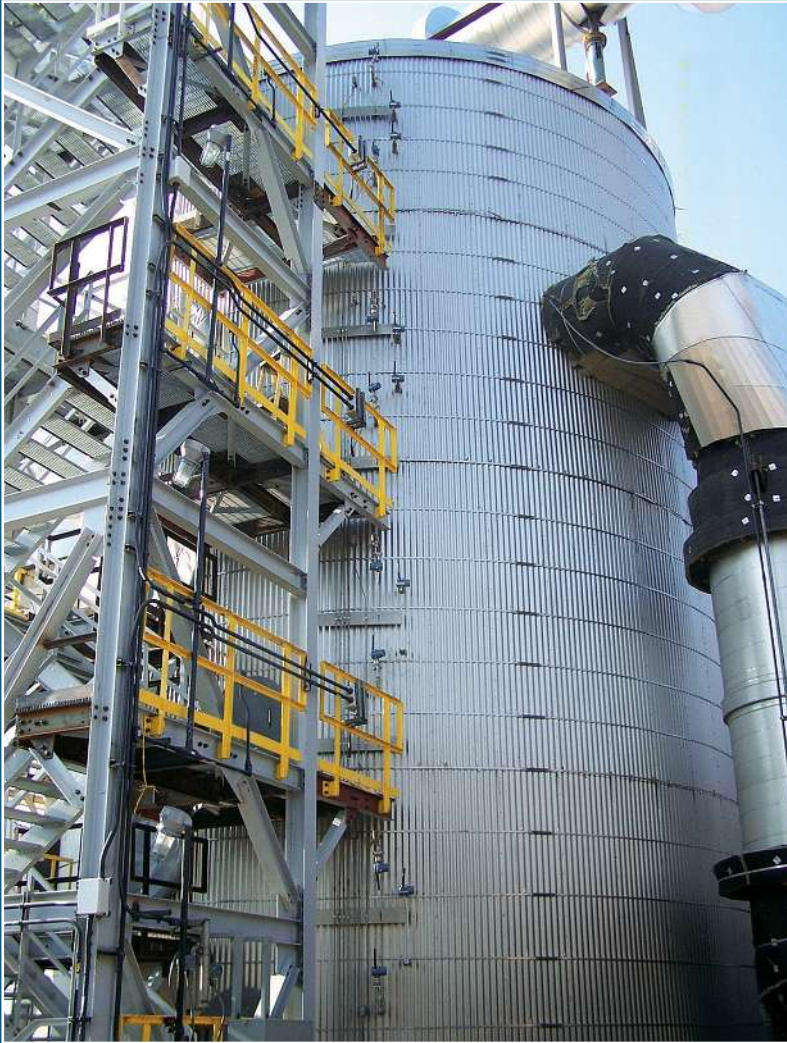
Picture: Emerson Process Management
